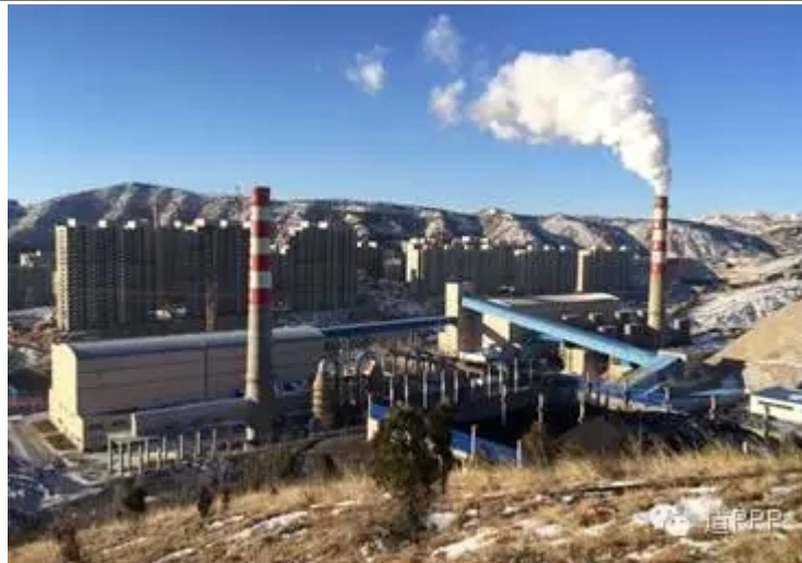
Overview of the Factory for Centralized Heating Project in Qiaoxi District
